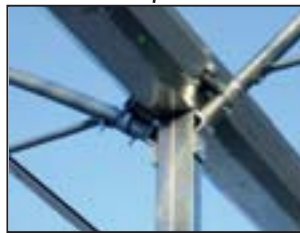
arc-column connection
